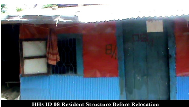
Photo 18: HH 08 before relocation in Polder-48
