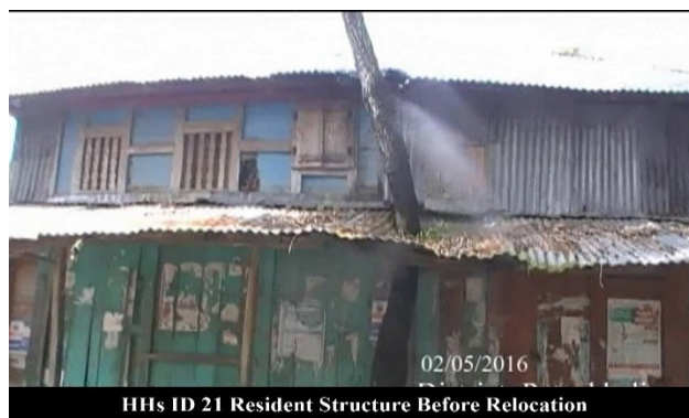
Photo 16: HH 21 before relocation in Polder-43/2C
