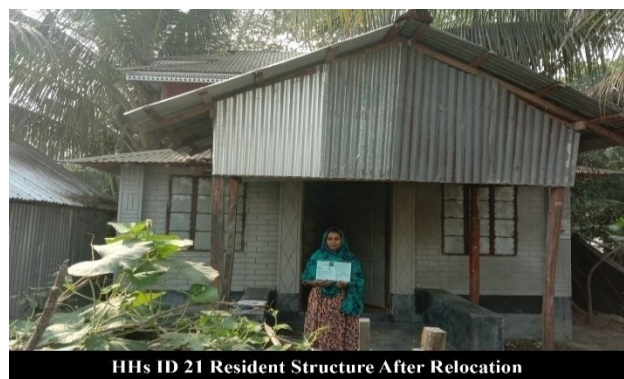
Photo 17: HH 21 After relocation in Polder-43/2C
